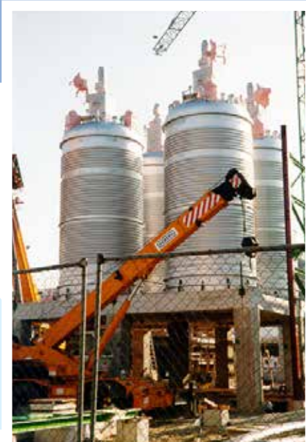
4 reactors 110 m 3 3 stages of GlasLock® agitators
